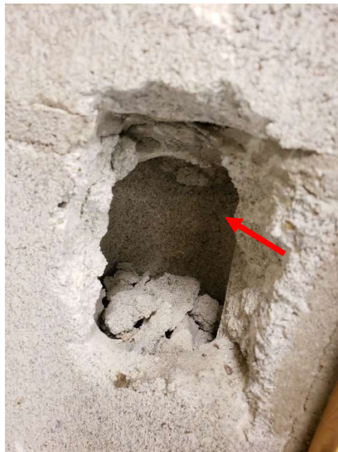
Photograph 2: Where observed, no vermiculite present within concrete block walls.
