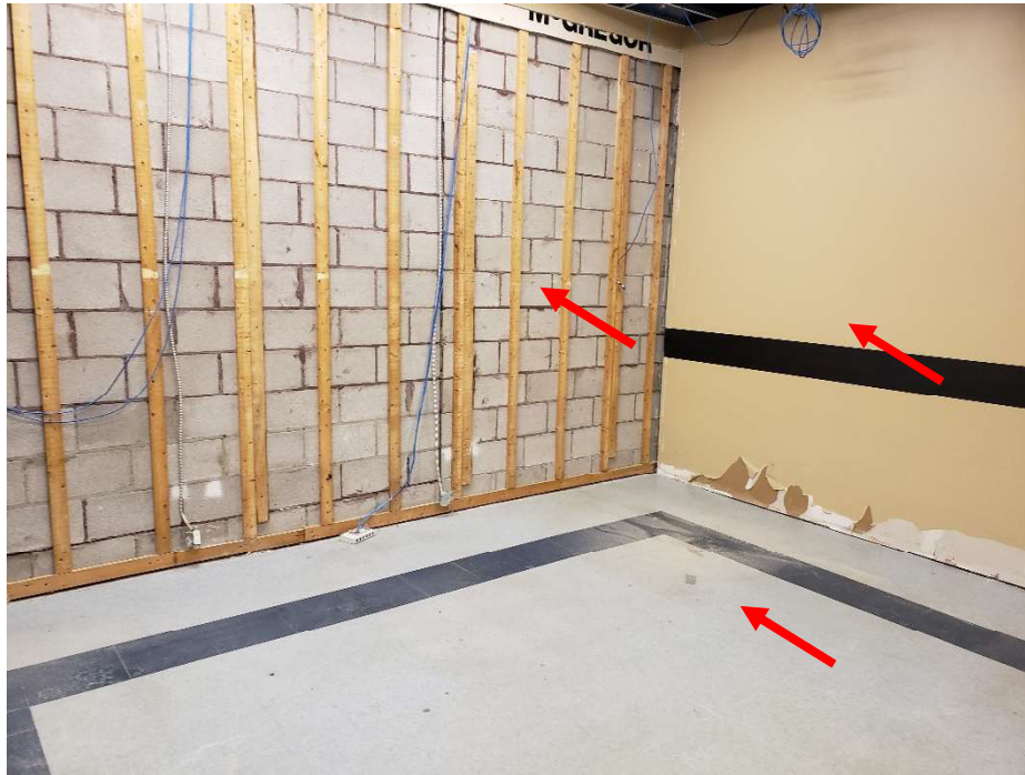
Photograph 1: Non-asbestos various 12"x12" vinyl floor tiles, drywall joint compound, and concrete brick mortar within former Classrooms, throughout Unit.
