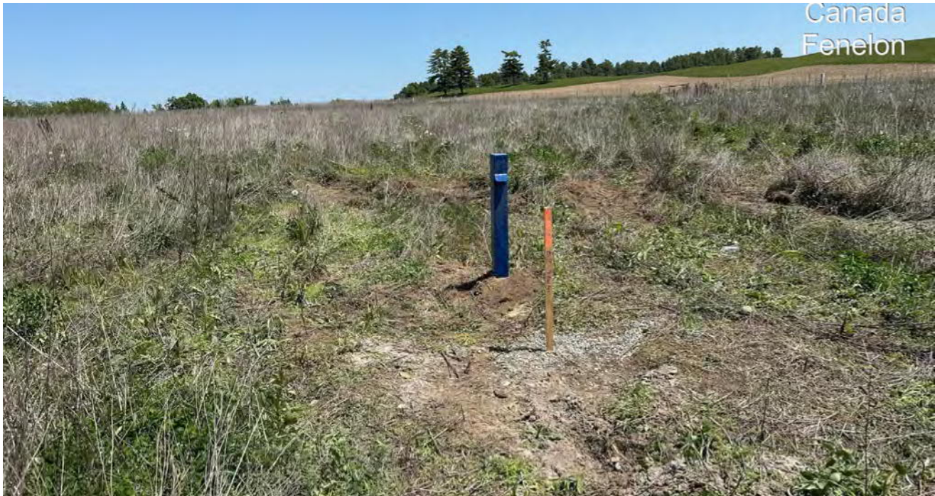
Photograph #3 – Looking east. Monitoring well is installed in the area of the proposed stormwater management pond (Borehole SWMP-02).
