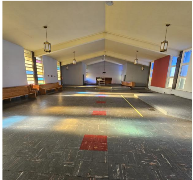
Photograph 2 – Nave Asbestos Floor Tile (9x9)
