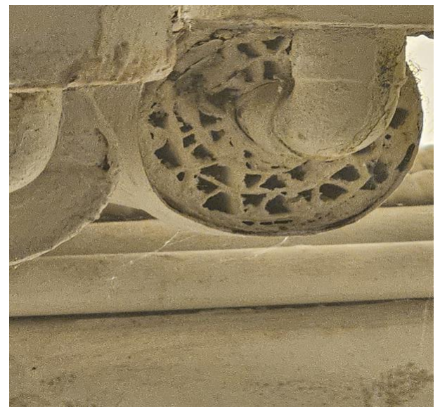
Photograph 4 – Photo of Asbestos Air Cell Insulation.
