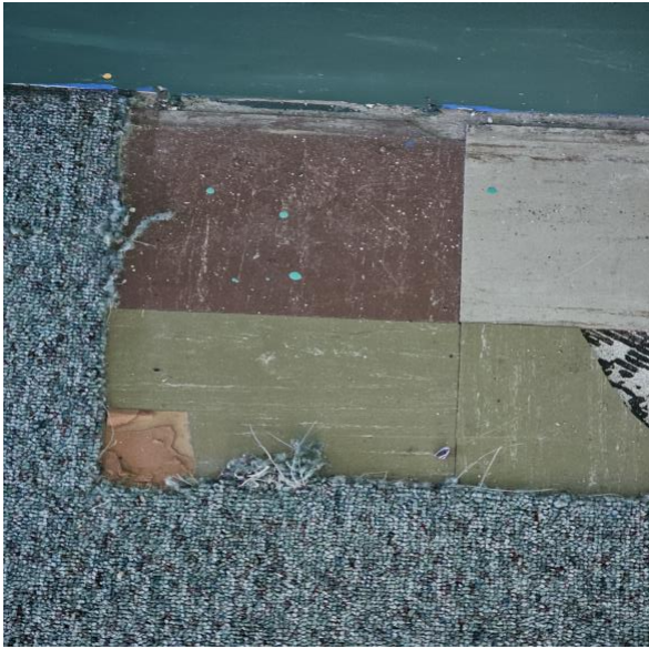
Photograph 1 – Basement Asbestos tile beneath the carpet.
